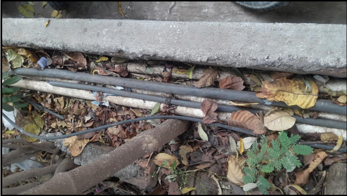
Drip Irrigation System
